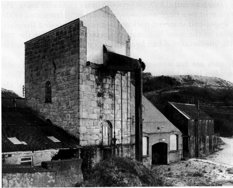
Fig. 3 Engine House, Goonvean China Clay Works, St Stephen in Brannel, Cornwall © copyright English Heritage
